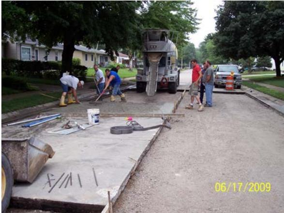
In May 2009 Excavation Plus was awarded the concrete street repair contract with a low bid of \$125,009. Concrete street repairs were made in the Everroad Park West neighborhood and Shagbark Court in Tipton Lakes. Excavation Plus removed and replaced 2745 square yards of concrete street, placed 893 tons of #73 stone and excavated 467 cubic yards of concrete and soil.
