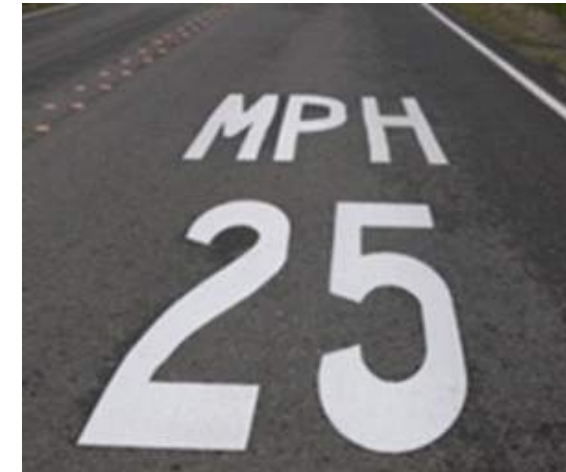
Speed Limit Pavement Legend
