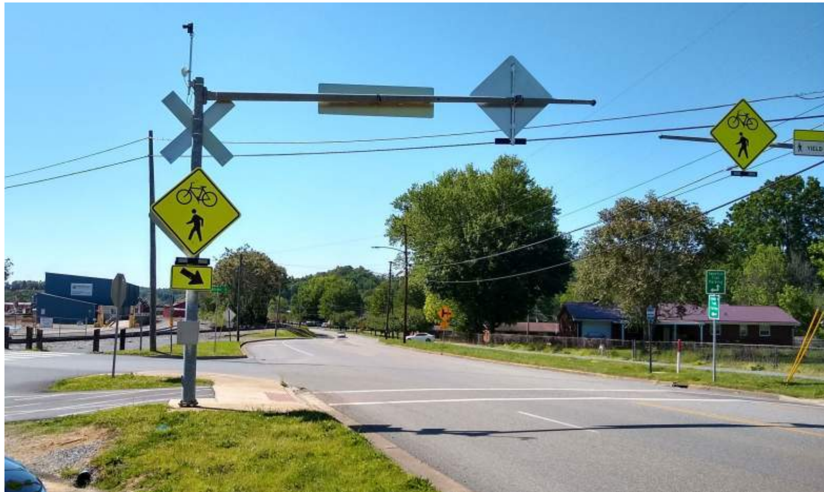
Trail Crossing Signs with RRFBs
