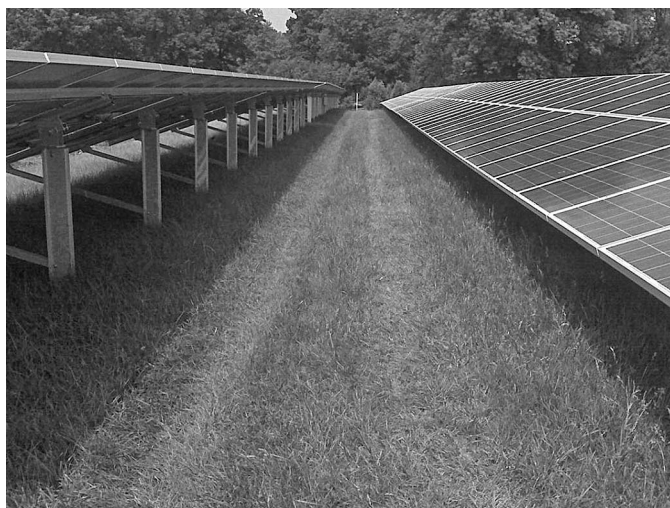
Fig. 1. Maintenance or “spacer” section between two rows of solar panels (photo by John E. Showler, reprinted with permission)
