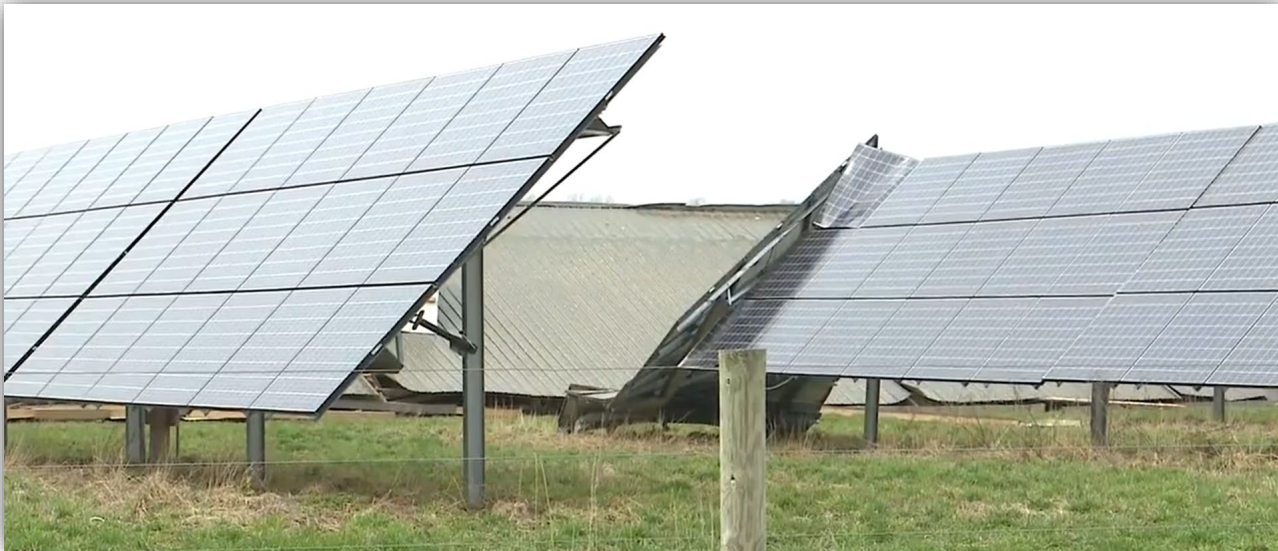
New Paris, IN April 2023 Straight-Line Wind Damage
