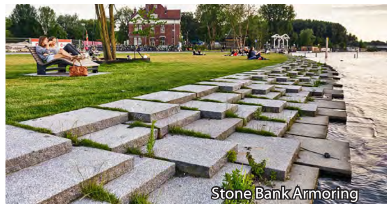
Limestone Retaining/Seat Walls
